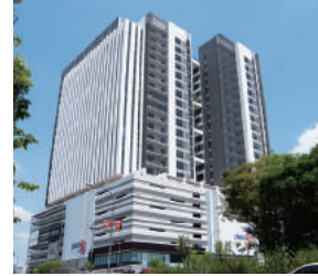
Malaysia Plaza 33 Office Block A
